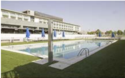
>>OCCIDENTAL HOTEL Outdoor pool
